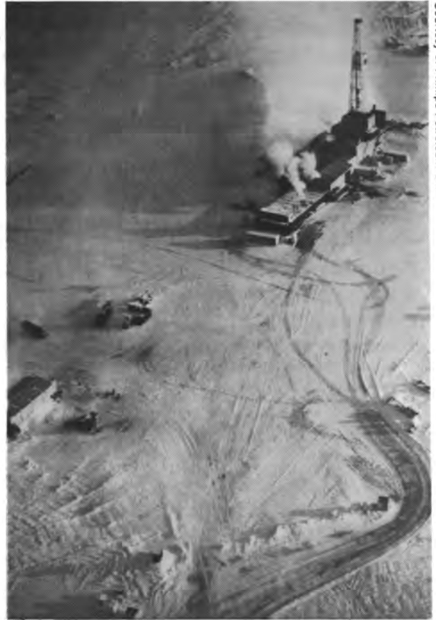
Fig. 1.2 – Man-made ice platform in deep water area of the Canadian Arctic Islands.
