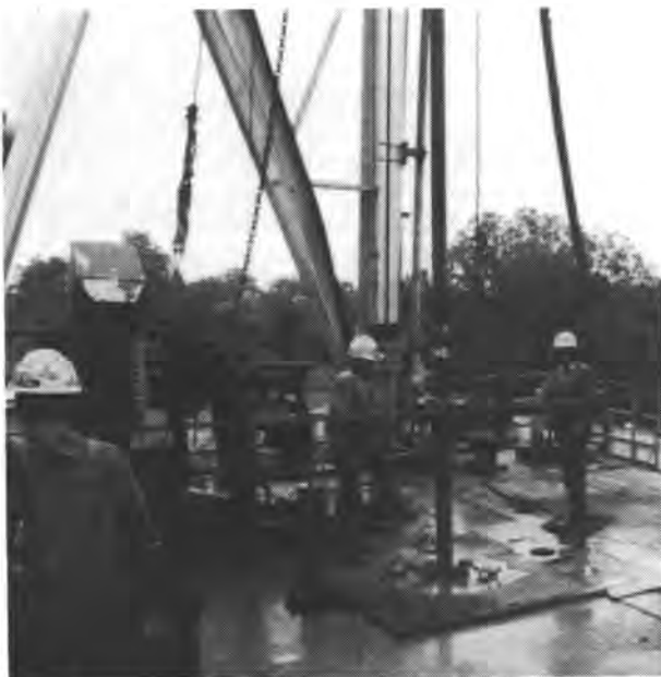
Fig. 1.21 – Tongs powered by chain to cathead.
